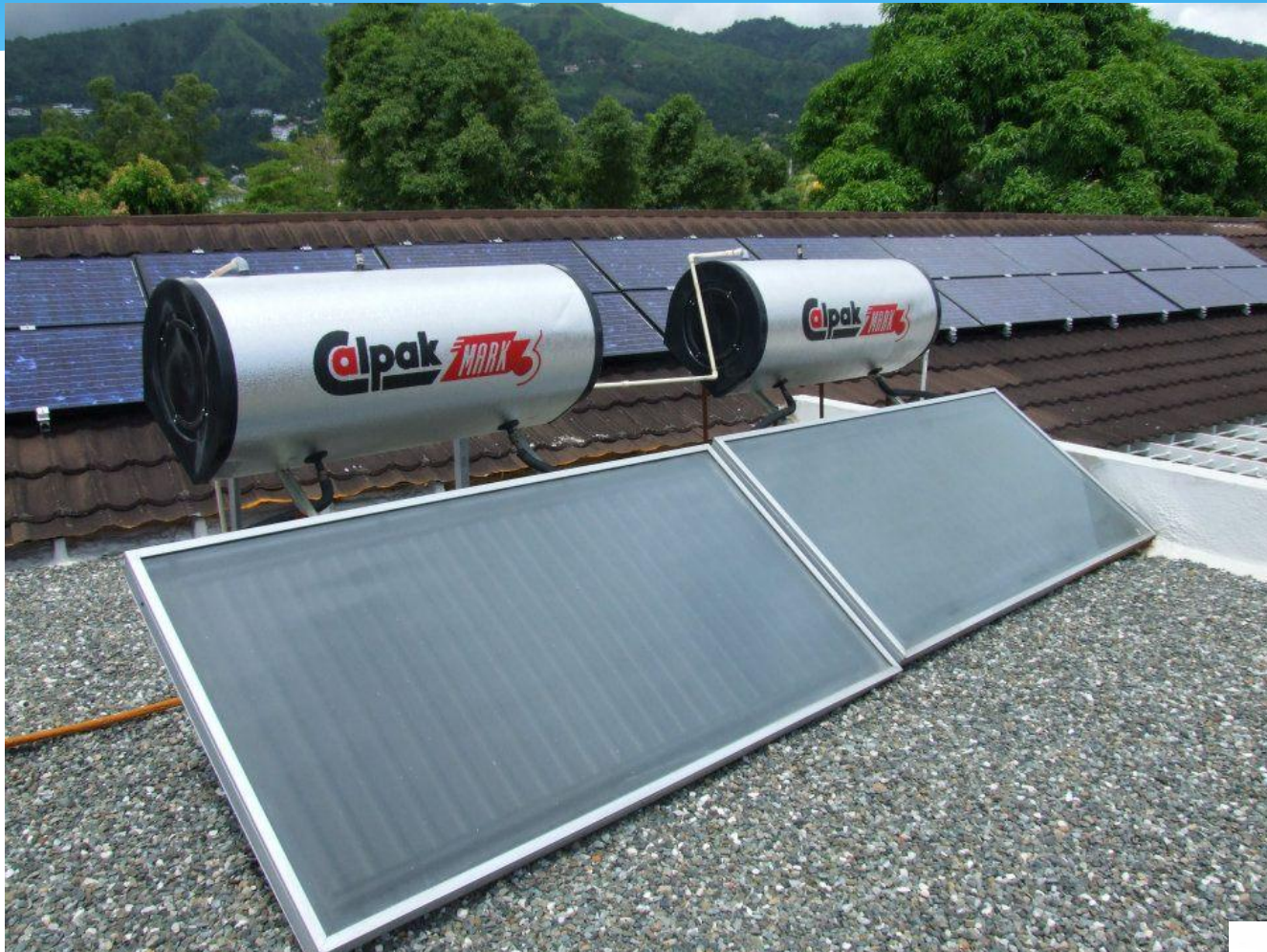
Solar PV and Solar Water Heating System installed at a Residence in St. Andrew
