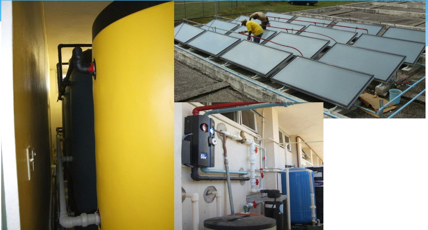
Solar Water Heater Installation at St. Ann's Bay Hospital
