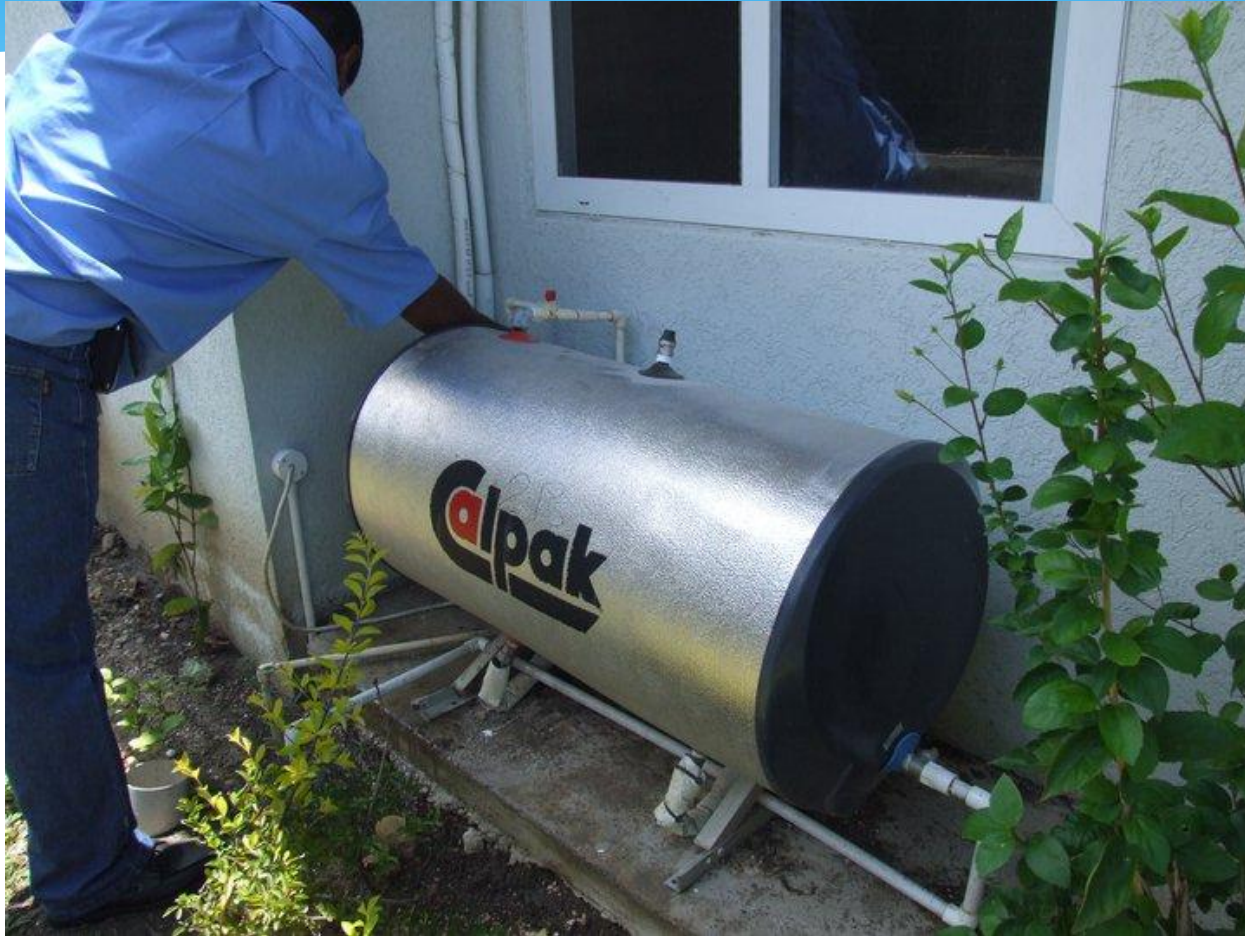
Solar Water Heater Installation at The Palms, Richmond, St. Ann
