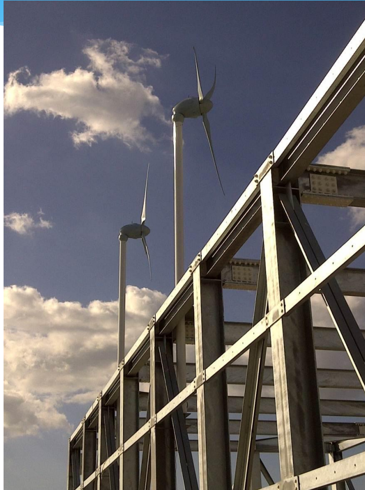
Skystream 3.7 Wind Turbines installed at Digicel Caribbean Headquarters, Downtown Kingston
